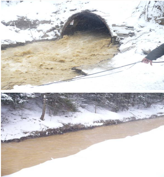
Figure 1 - Water outflow from Nová štôlna and view on the dirty stream
