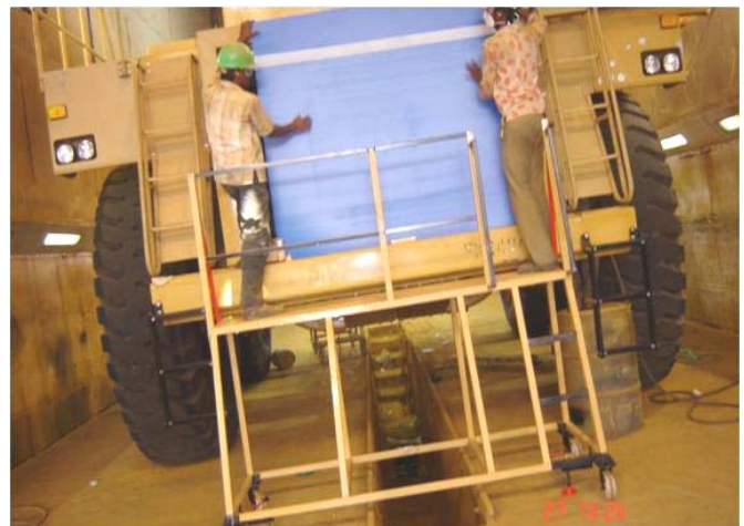
Figure 9. Masking with safety trolley - operator risk eliminated
