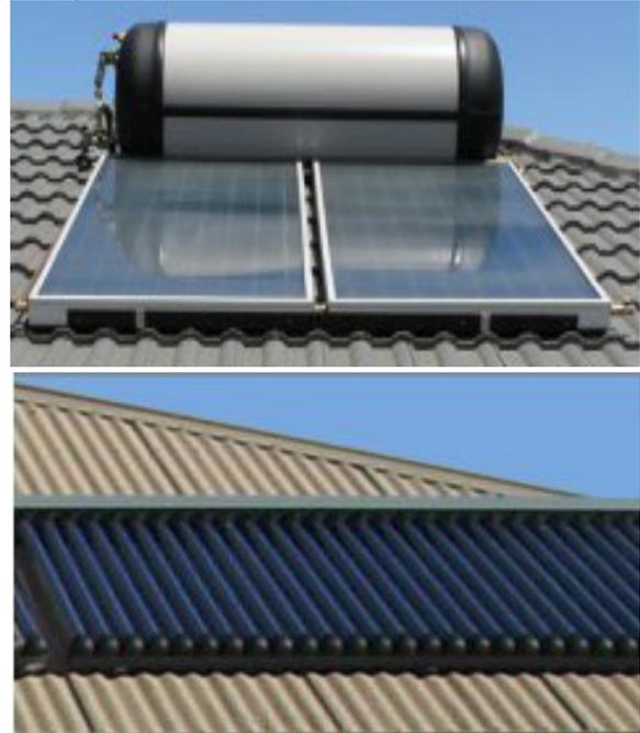
Figure 1. Flat panel (left) and evacuated tube collectors
