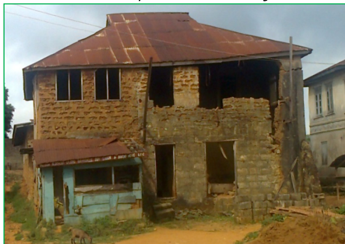
Figure 1: Picture of collapsed building from red sand blocks
