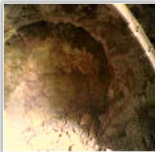
Figure 4: Blasting result in the gallery
