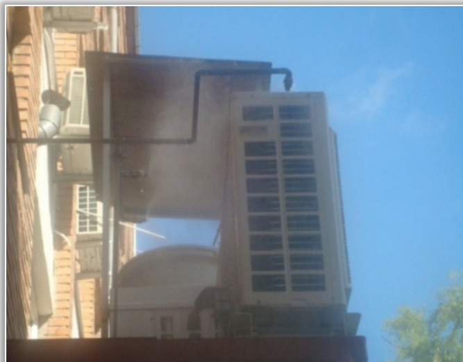
Figure 4. Water spray system for condenser cooling
