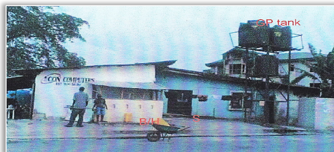
Figure 3: Borehole located 4 metres away from septic tank with GP tank on top along Ikpa Road
