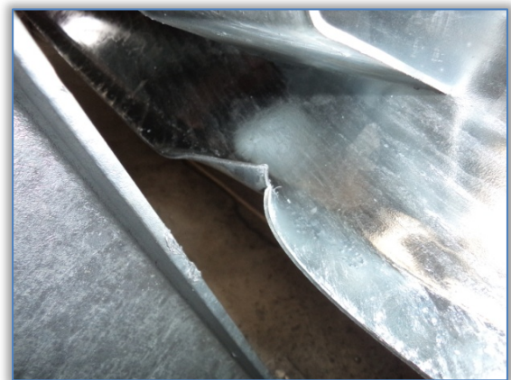
Figure 10: Slide broken in the area of pillar
