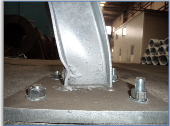
Figure 9: Pillar deformed on the edge
