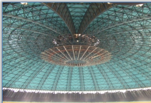
Figure 3. Internal view of the dome
