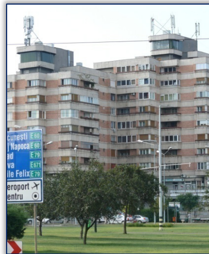
Figure 7. GSM Antennas on living block in civic center
