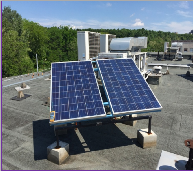
Figure 3 -Solar panels used for the measurement
