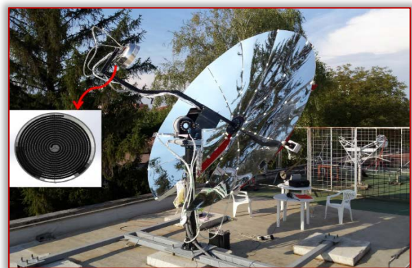
Figure 1. The examined solar dish collector
