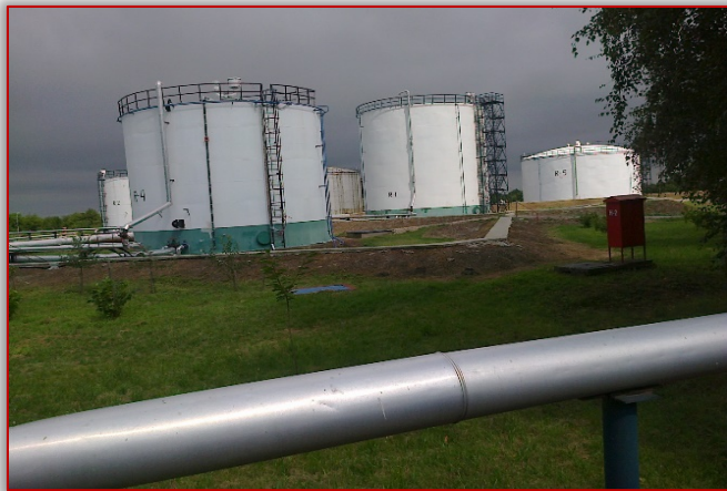
Figure 3. The appearance of the oil collecting station
