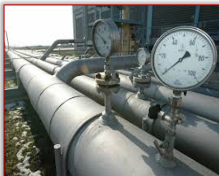
Figure 5. Appearance of the above-ground oil pipeline
