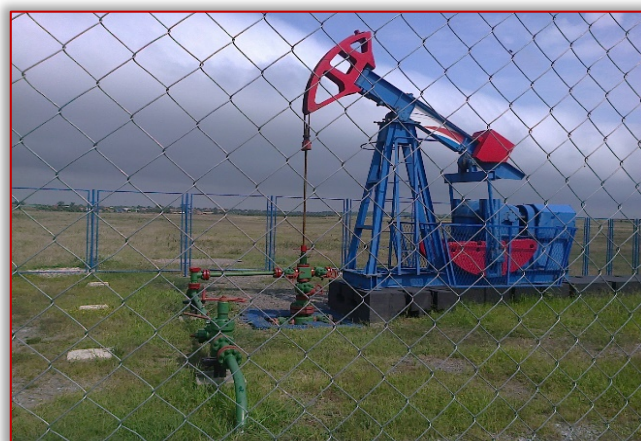
Figure 2. The appearance of the pump well
