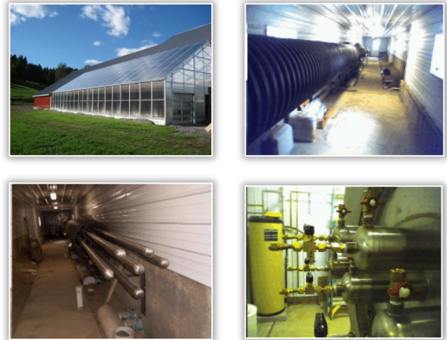
Figure 4 – Industrial system implemented at Diamond Hill Custom Heifers
