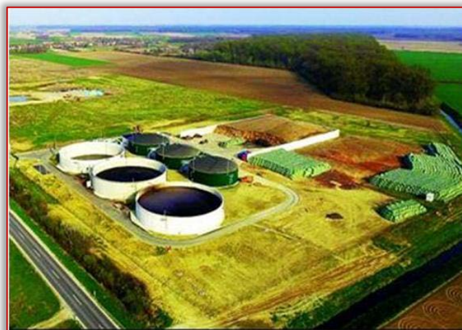
Figure 4. Biogas power plants (2 MW) "Biointegra" Slatina, Croatia [8]
