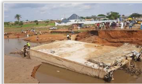
Figure 3. Alagbado bridge along Foma-river washed away by the flood
