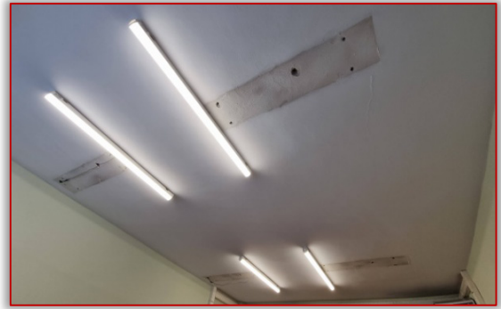
Figure 14. New LED lighting immediately after installation
