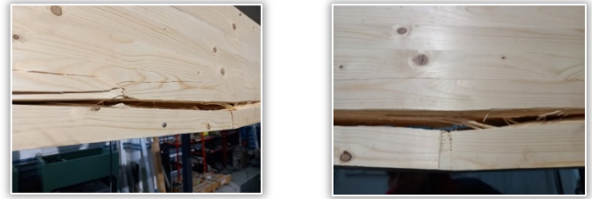
Figure 4. Failure patterns of the tested specimen Type 1 (No Polymeric reinforcement)
