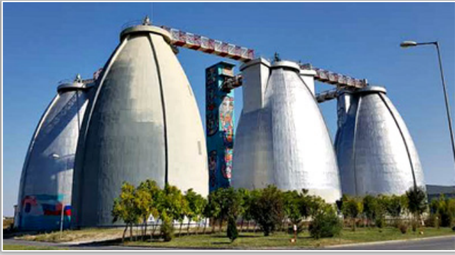
Figure 1. The Bucharest Municipality Water Purification Center
