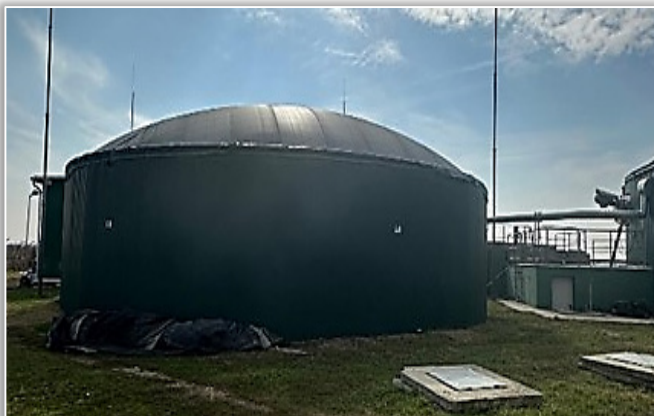
Figure 3. Fermentation tanks: the sludge reservoir is coupled with the gas reservoir in the same construction
