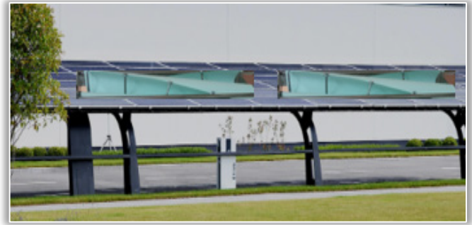
Figure 9. Photovoltaic canopy (bus station) with wind generators (turbine is a photovoltaic panel, too).
