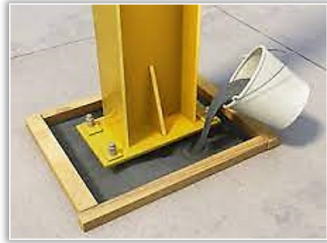
Figure 8. Cementitious grout injection
