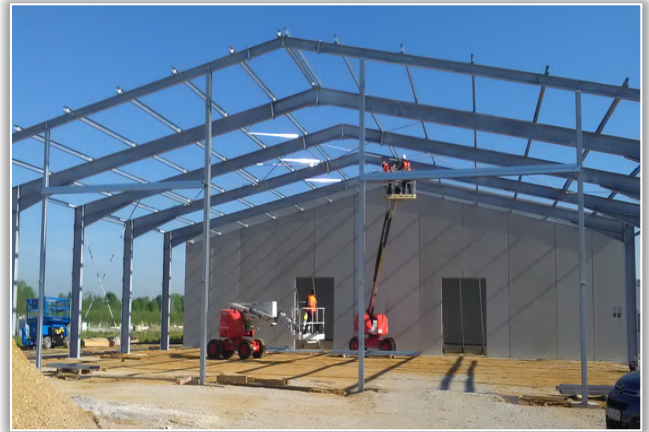
Figure 3. Steel structure of the hall [1]
