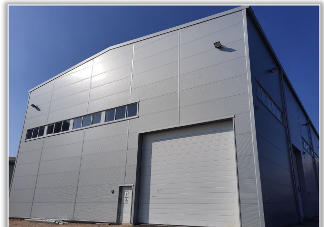
Figure 5. Facade wall made of sheet metal "sandwich" panels [1]
