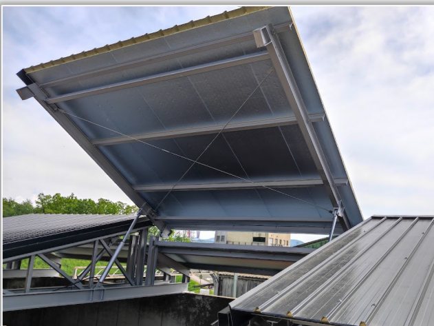
Figure 2. Retractable steel roof with "sandwich" panels [1]
