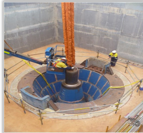
Figure 7. Replacement of the Main Shaft
