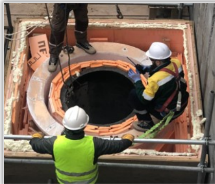
Figure 8. Replacement of the Eccentric Bush
