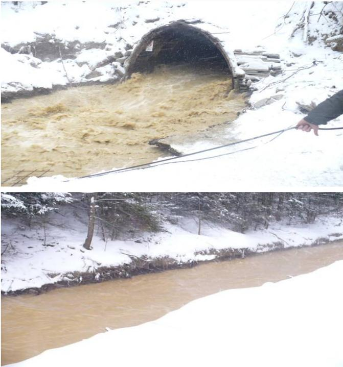
Figure 1 - Water outflow from Nová štôlniča and view on the dirty stream
