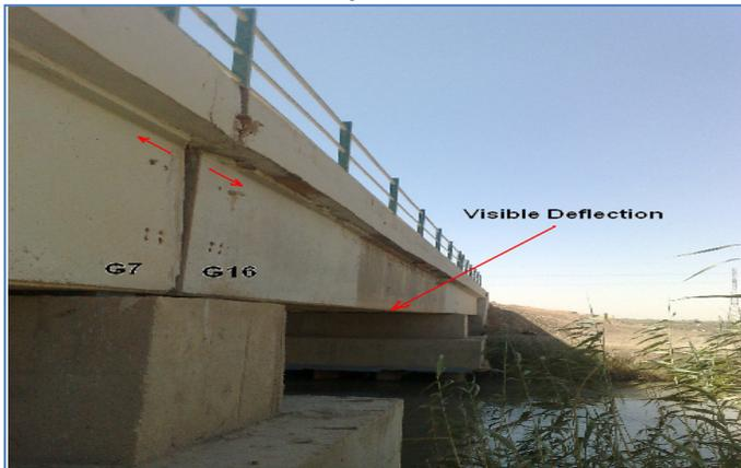
Figure 5. Visible mid span deflection at the right side of the intermediate panel
