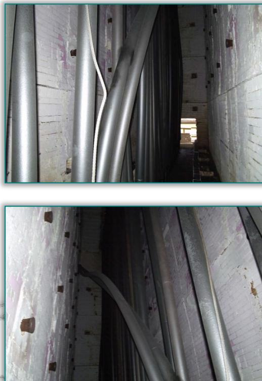
Figure 2. Pyrolysis furnace radiant zone – consequence of a high creep rate
