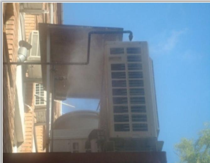
Figure 4. Water spray system for condenser cooling
