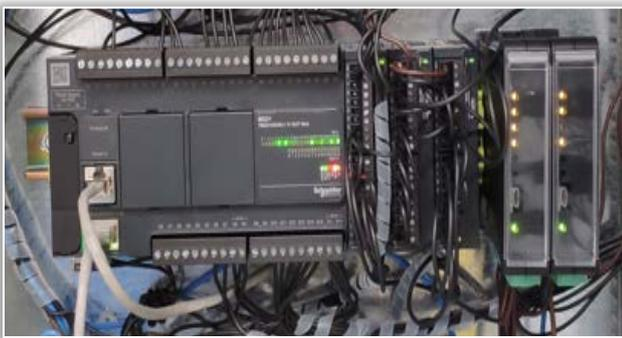
Figure 3. PLC Schneider Electric M221 with analog input/output modules and the proportional controllers located in the electrical cabinet
