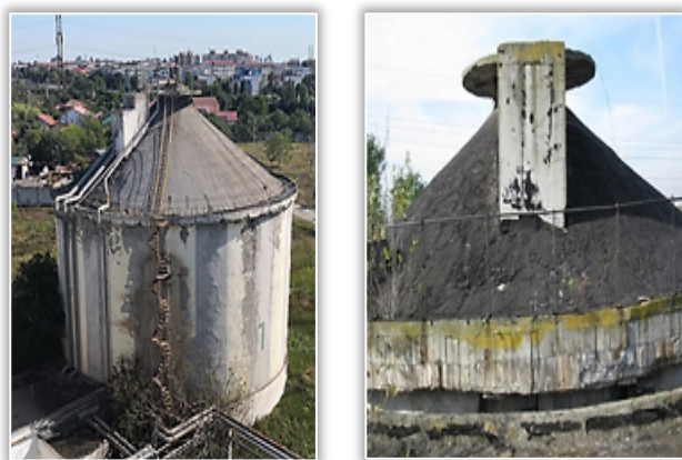
Figure 6. Cylindrical-conical fermentation tanks with cracked roof dome
