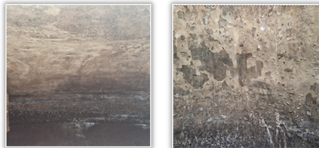
Figure 8. Chemical attack on the inner surface
